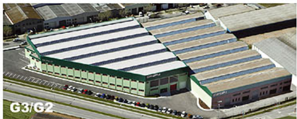
FACTORY GIRBAU 2: heavy-duty laundry equipment (batch washers, presses, dryers, conveyors, etc.)
