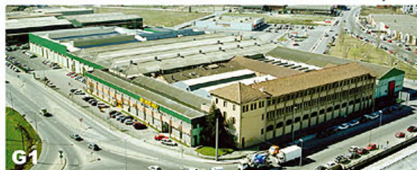
FACTORY GIRBAU 1: washer extractors and flatwork ironers
